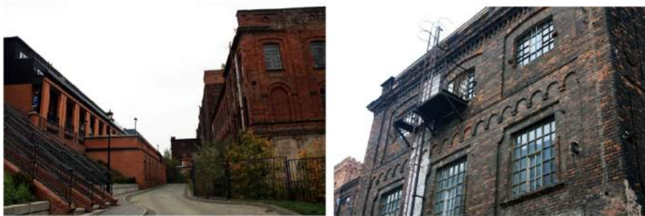
Fig.5 On the left: A part of Scheibler lofts redeveloped and in contrast the decaying parts
