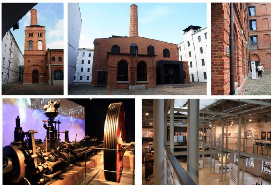
Fig. 8. The current state of the object The Geyer Factory, after revitalization White Factory
